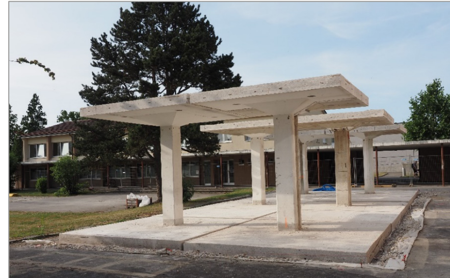
rebuilT Pavillon associatif (Ecublens, CH, 2023)
